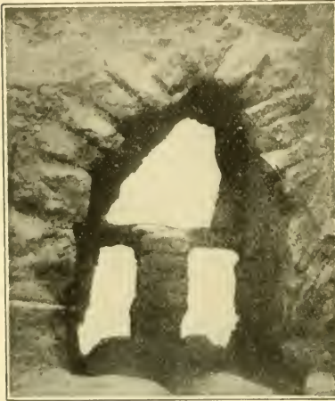
THE OLDEST ARCH KNOWN (about 4000 B.C.). This vaulted drain was discovered a few years ago fifteen feet below what had long been supposed to be the earliest remains of Babylonian civilization. It seems to have been part of a highly complex drainage system in a crypt of an ancient temple. The arch is two feet high. The clay pipes, whose forms can be seen dimly on the bottom, are eight inches in diameter, and lie in two-foot joints.
